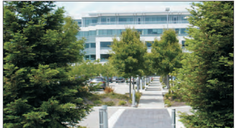
View of southern portion of Parcel 1A from Iron Horse Trail.
